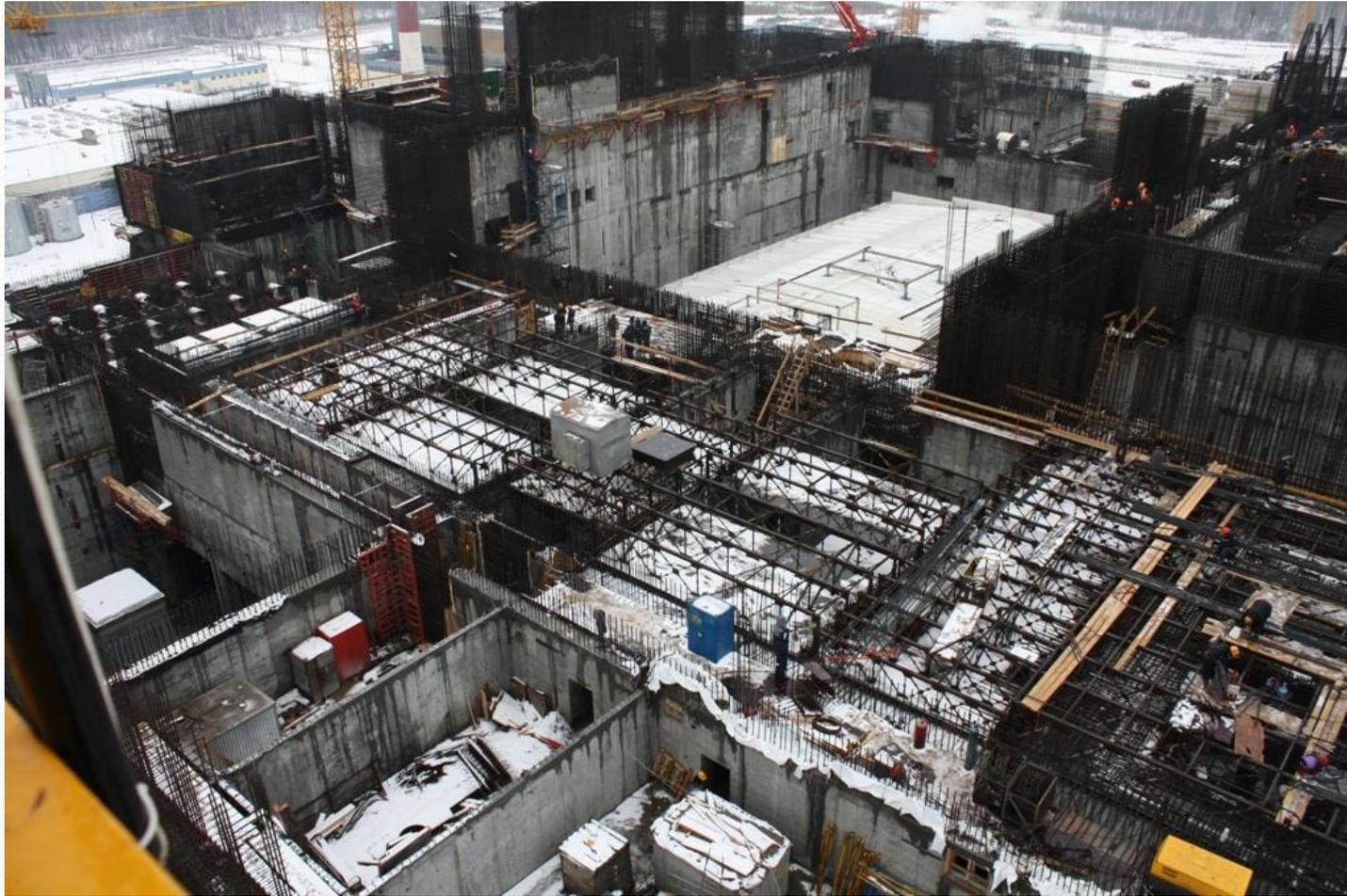
**Bird's-eye view of the steam generator compartment of the main building**
